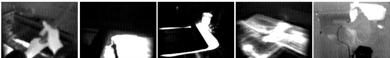
Figure 2: Practical application of collaborative Computer Mediated Reality: (leftmost) First person perspective as captured by the EyeTap device. Author's hands are visible grasping the mop. (left of middle) Mop and hot asphalt as viewed through bearer's right eye. (middle) After mopping hot asphalt onto the roof surface, a base sheet is rolled down (bucket of hot asphalt shows as white in the upper right area of the frame). (right of middle) The thermal EyeTap is useful for "seeing through" the top layers of felt or fiberglass, to determine heat flow underneath. (rightmost) The kettle (upper right of frame) shows up as white (approx. 500 degrees) whereas the propane cylinder (bottom of frame) and the propane hose supplying it show up as black, because the cylinder and hose are cold due to the expansion of the propane gas. The thermal EyeTap was also useful when the kettle caught on fire because of its ability to see through smoke. Kettle fires are easy to extinguish (simply by slamming the lid shut) if the kettle can be seen through the thick black smoke given off by the burning asphalt.
