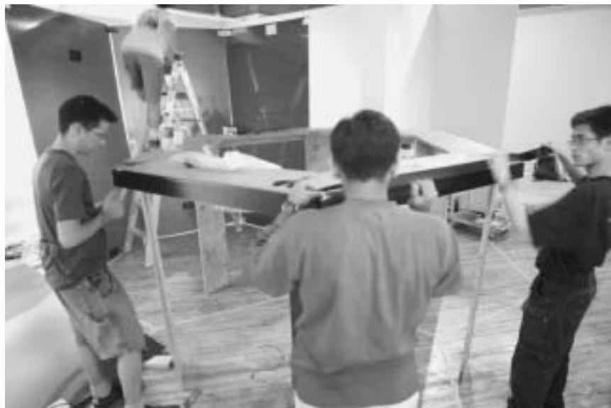
Fig. 2. Building the hexagonal-shaped countertop and moving it into position so that six walls made of darkly tinted bulletproof "glass" (darkly smoked lexan polycarbonate) can be built around it, to form the central room of the seven rooms depicted in Fig. 1. (© Steve Mann) Three of these walls are being assembled behind the stepladder shown in the background and will later be moved forward and joined to the other three walls to complete the central guard tower.
