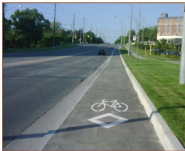
Figure 4.27 – Raised Cycle Track, City of Guelph
