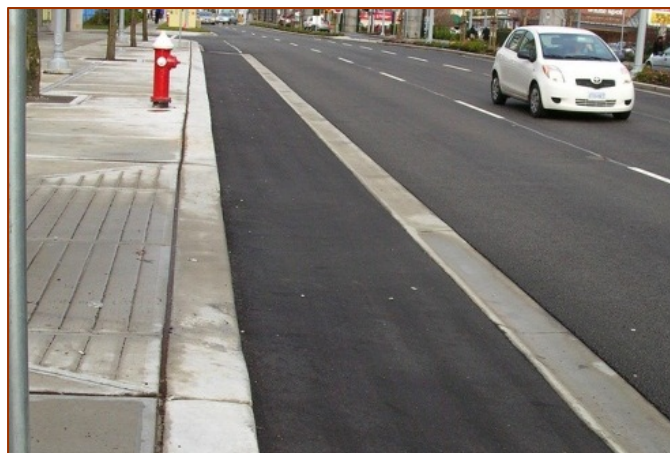
Figure 4.30 – Asphalt Raised Cycle Track Source: Stephen Rees (Flickr), 2010
