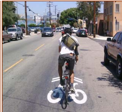
Figure 4.2 – Shared Roadway with Optional Sharrows
