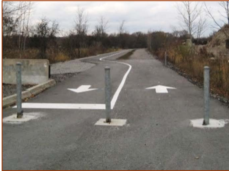
Figure 5.19 – Bollards restrict unauthorized motorized vehicles from accessing the off-road cycling facility, Orillia, Ontario
