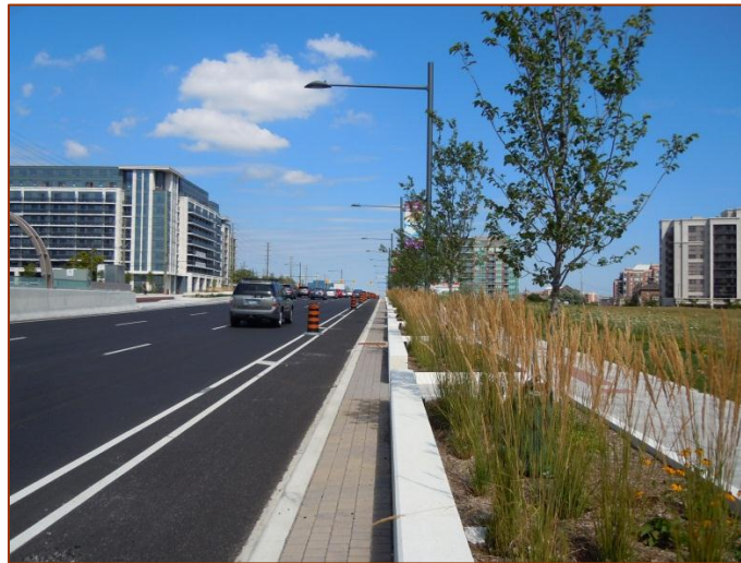
Figure 4.21 – Bicycle Lane and Vehicular Travel Lane separated by a painted buffer, York Region
