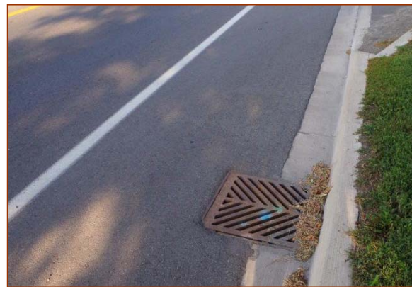
Figure 4.59 – Example of a Drainage Grate with Herring Bone Openings and Concrete Gutter
