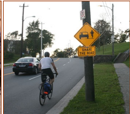
Figure 4.3 – Shared Roadway with Wide Travel Lane
